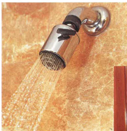
▲ Water restrictors installed in showers can reduce water consumption by around 15 per cent. 在灑水器上安裝調節器，可減少用水 15%。
